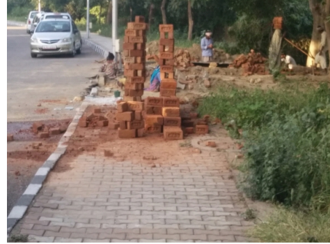
(b) Debris over the sidewalk
