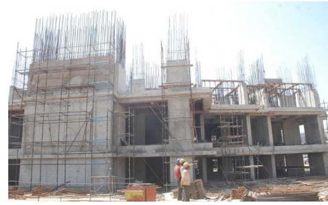
(a) House under construction
